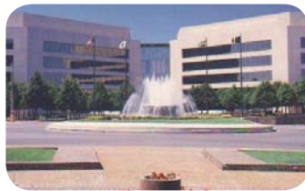
St. Clair County Courthouse, Illinois
