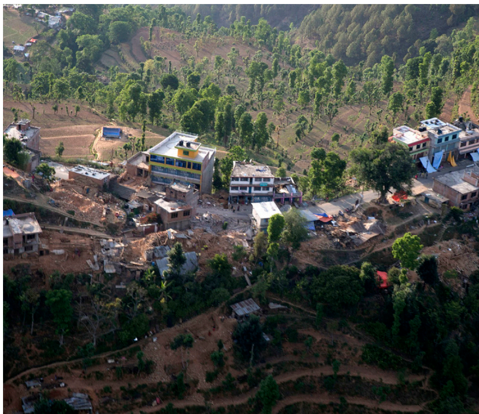
Caption: Photograph of the destruction in Nepal taken from a US Army helicopter Source: Lance Cpl. Mandaline Hatch
