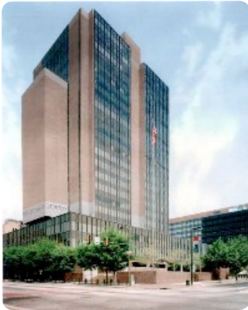
U.S. District Court, Eastern District of Pennsylvania
