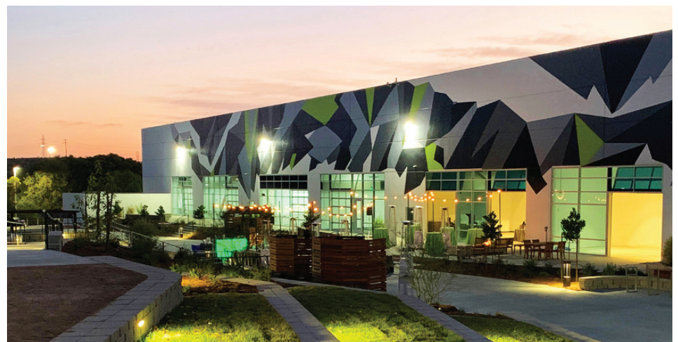
ATEC New Headquarters back view / Courtesy of Alphatec Holdings, Inc.
